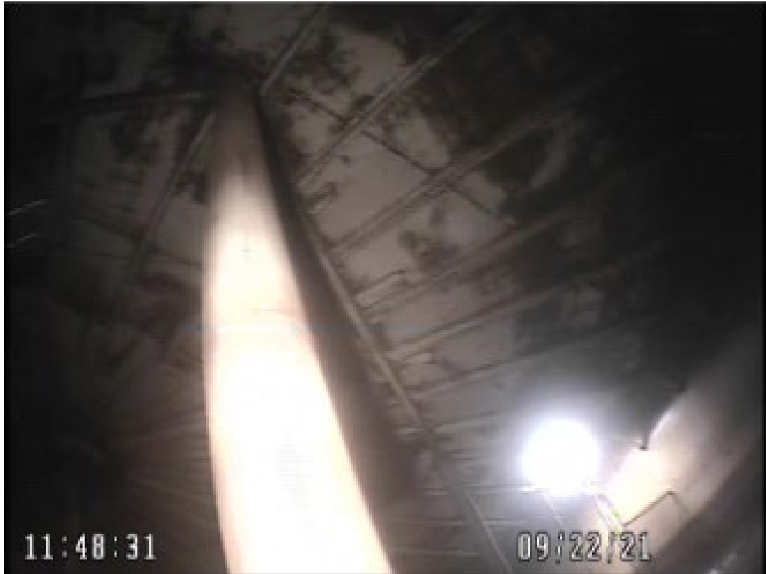
Significant rust on interior tank surfaces
