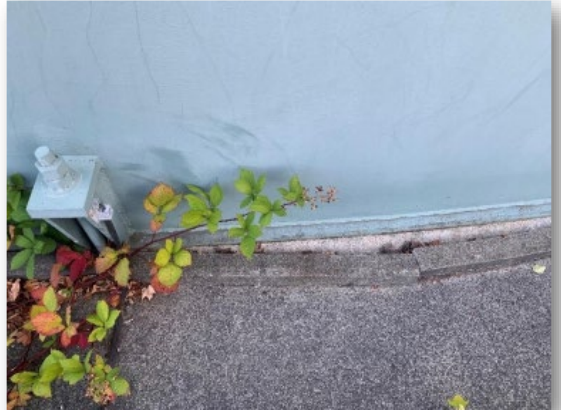
Damaged concrete curb
