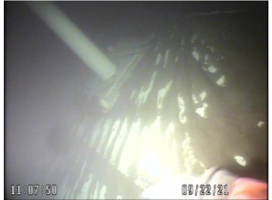
Significant rust on interior tank surfaces
